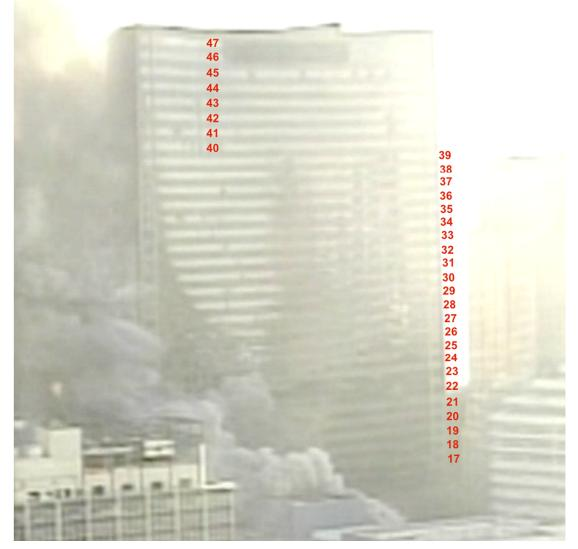
Figure 4.25: Floors 17 to 47 falling uniformly as a unit (CBS).
