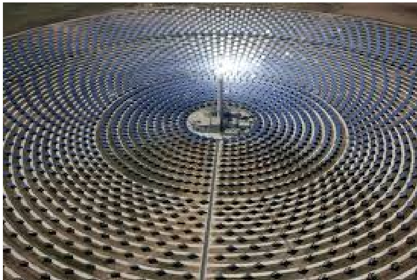
Figure 7.11: A solar thermal power plant. Arrays of heliostatic reflectors concentrate the sun's rays onto molten salt in the tower. The plant produces electricity at night because the salt remains hot..
