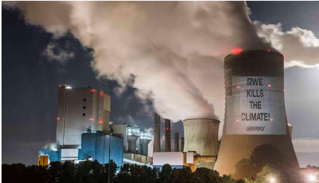
Figure 7.6: A coal-fired power plant.
