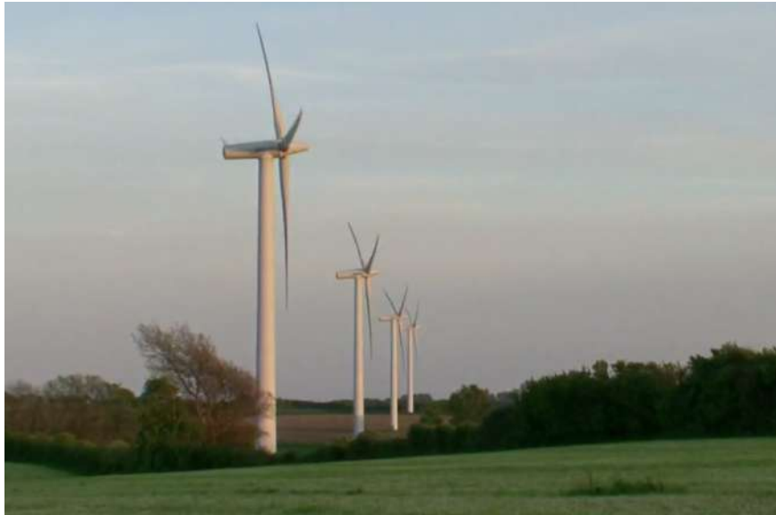
Figure 7.16: Wind turbines on the Danish island of Samsø The island was the first in the world to achieve 100% renewable energy.
